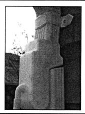
Install at downspout elbow.
